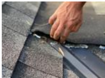
Crack or tears
