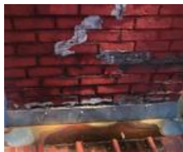
Cracked flashing
